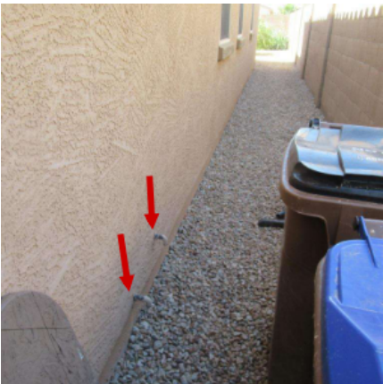
Image 5.1.1 Discharge Pipes on West Wall
