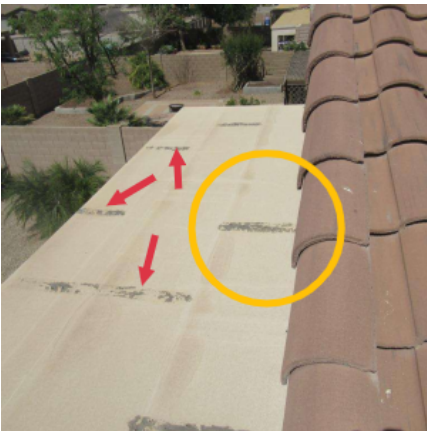
Image 2.2.2 Peeling coating from joints on patio roof
