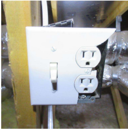
Image 3.4.1 Broken Outlet Cover
