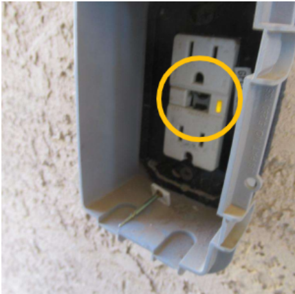
Image 3.3.3 Broken GFCI Test Button
