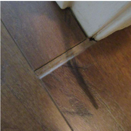
Image 6.1.1 Hardwood Flooring Gap - Master Bdrm Entry
