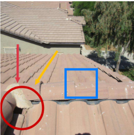
Image 2.2.1 Roof tile has slid out of place - NE Corner of Home
