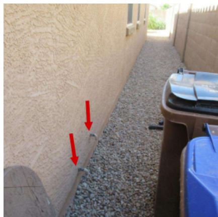
Image 5.1.1 Discharge Pipes on West Wall
