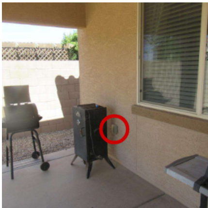
Image 3.3.1 Broken GFCI Location
