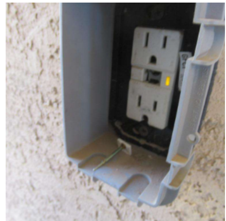
Image 3.3.3 Broken GFCI Test Button
