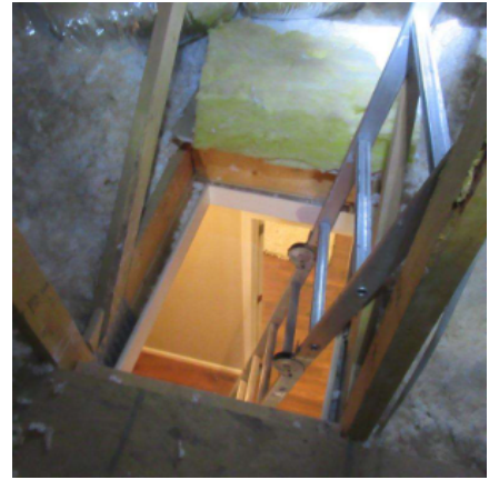
Image 3.4.3 Entry to Attic
